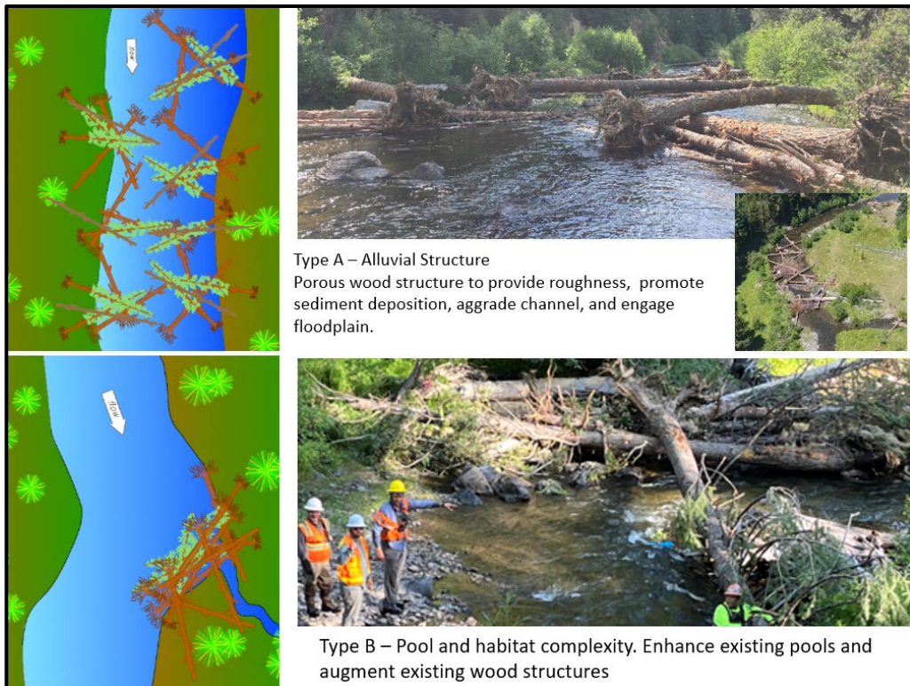
Figure 7. DESIGN VIEW (left) AND CONSTRUCTION PHOTOS (right) OF WOOD AND BOULDER STRUCTURE TYPES USED ON THE MUGRR PROJECT
